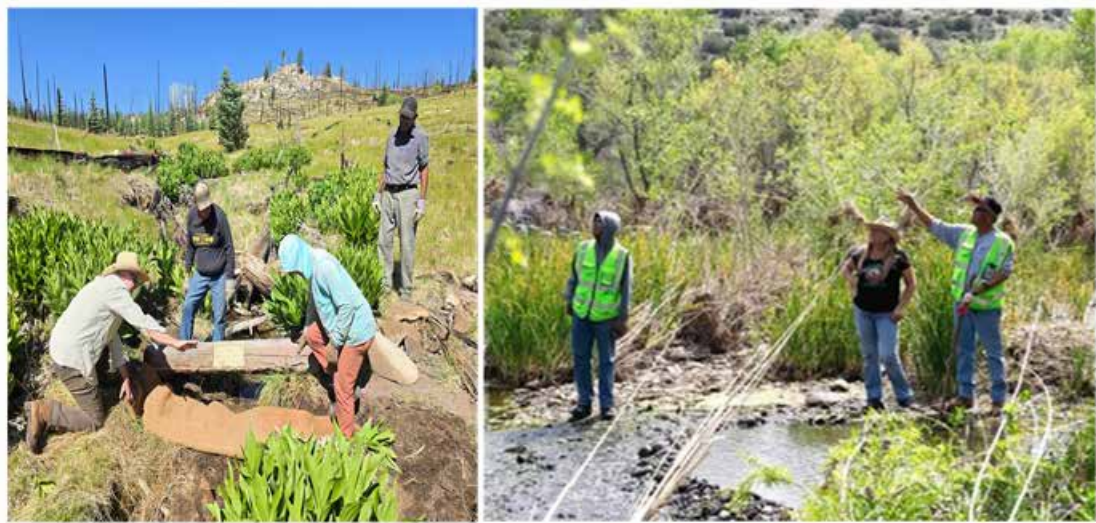
Figure 4.2a & b. (a) The San Carlos Apache Tribe Restoration Crew and the Taproot Collective installing erosion control structures as part of a spring restoration project on Mt. Graham in Coronado National Forest, one of the three National Forests that shares a boundary with the Reservation. (b) The San Carlos Apache Tribe Department of Environmental Protection installed NIDS to protect sacred water and springs in partnership with the USGS on the Tribal Land Vegetation and Watershed Modeling project.
