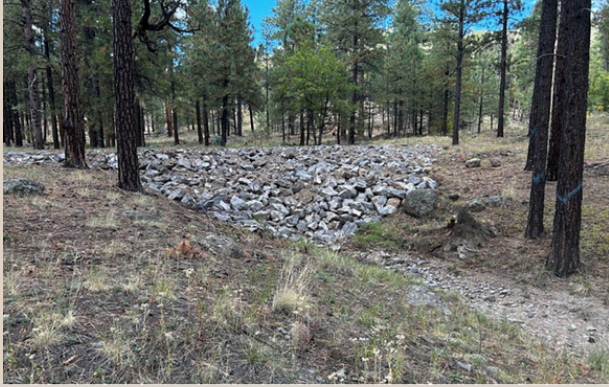
A pond-and-plug structure, an example of ORE in flood water management. (Source: Gupta et al, 2026)
