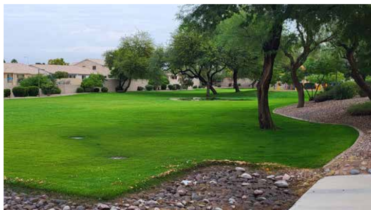
Figure 4. A retention/detention basin with drywells used as a flood control strategy to capture and direct stormwater for recharge in Chandler, AZ. Photo: Dr. Tianfang Xu, ATUR Urban and Recharge teams, ASU.
